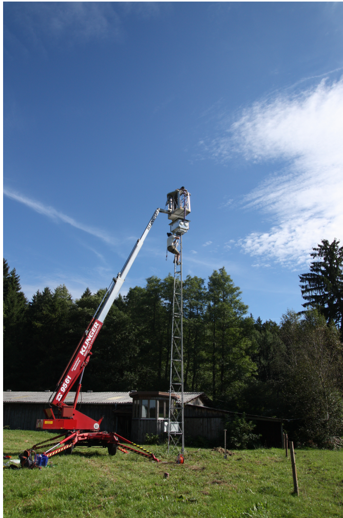
Figure 3.4 – Picture of installation work at the TERENO test site Fendt .
