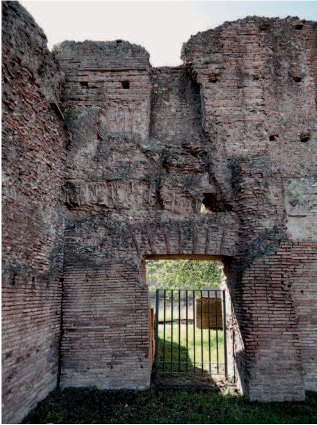
Figure 5 Entrance to room 533S, seen from the west: The existing entrance is a later reduction of a wider opening from the original building phase. The changes can be deduced e.g. from the remains of the relieving arches. Photo L.C. Götz.
