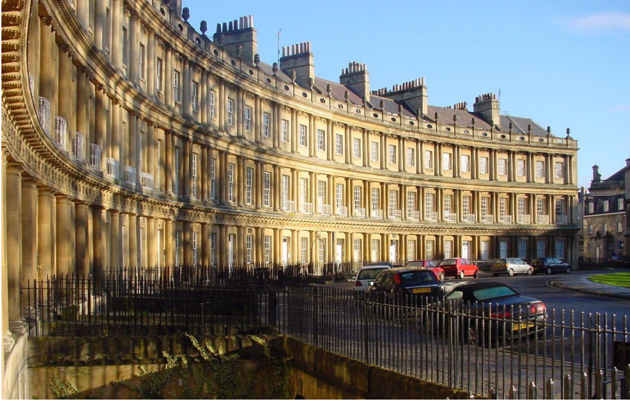
(A) Royal Crescent Townhomes, Architect: John Wood the Younger, Bath, England
