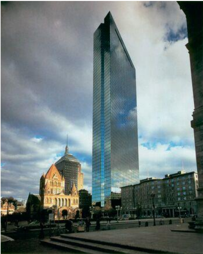
(F) John Hancock Tower, Architect: Henry N. Cobb, Boston, Massachusetts
