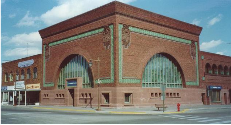
(E) Owantonna Bank, Architect: Louis Sullivan, Owatonna, Minnesota
