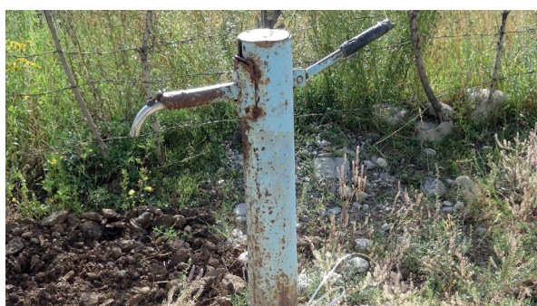
Fig. 4: Blue well with a modified handle and water outlet
