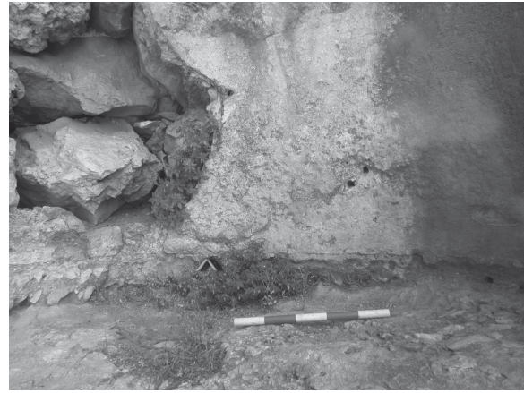
14. Small, southern (?) apse, looking east. The apse was plastered and paved with mosaics. Arrow marks level of mosaic floor (photo by authors).
