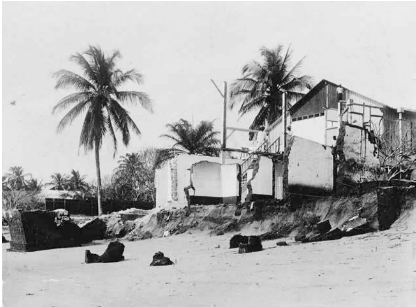
Fig. 1: Material and moral damage: Northern German Mission Society's house in Keta (Ghana) after a storm in 1914 (Picture courtesy of Bremen State Archive, StAB 7.1025-Fotos-0788)
